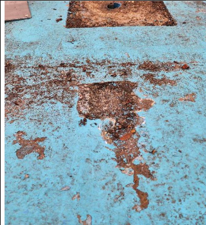
Photo 3: Further Screed breakdown
