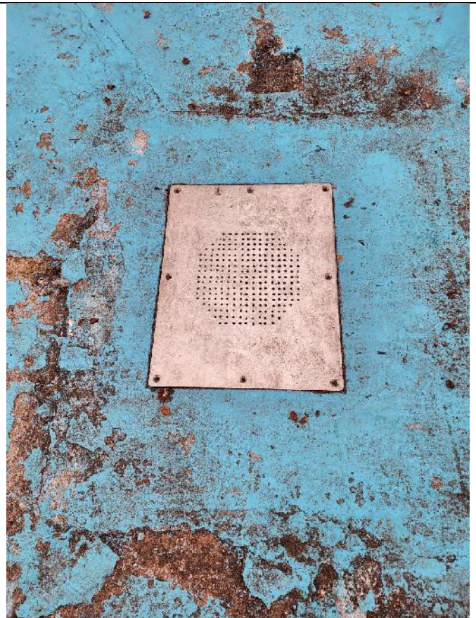
Photo 10: Central drain with cover over – no fixings present
