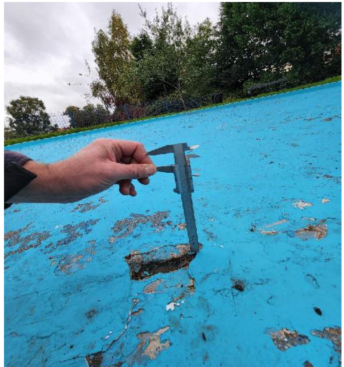
Photo 2 – Deepest Screed breakdown 20mm
