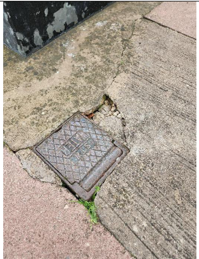
Photo 12: Cracked concrete and dropped levels – Hazardous to pool users
