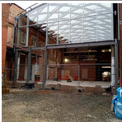
Glazing installed to courtyard
