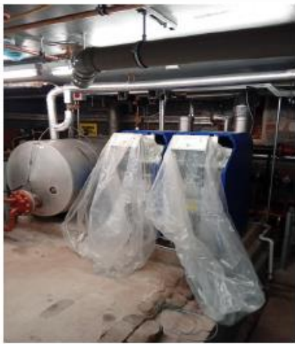
New Boiler installed
