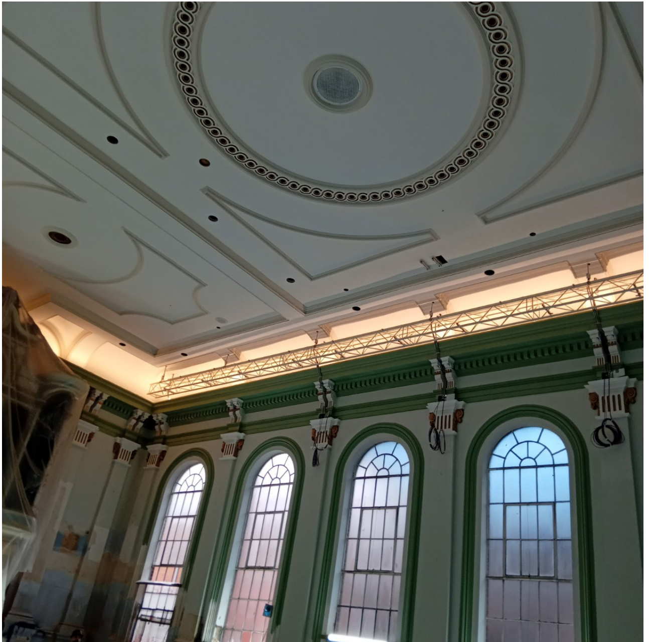
Installing new LED feature lighting.
