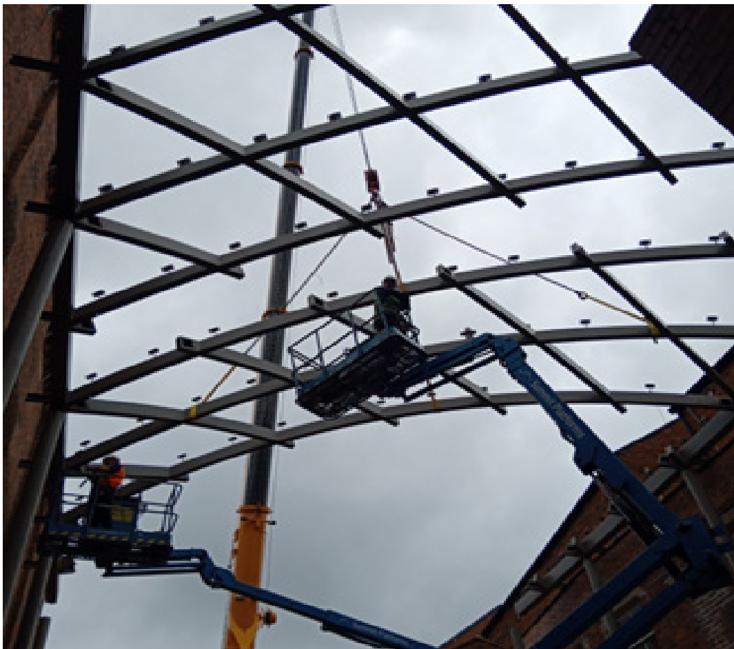
Crane lifting roof into place
