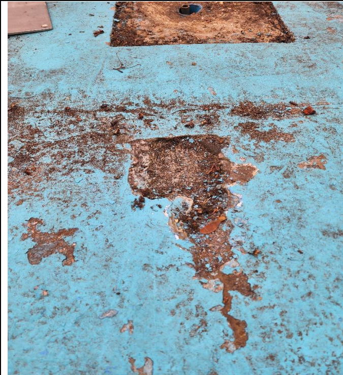
Photo 3: Further Screed breakdown
