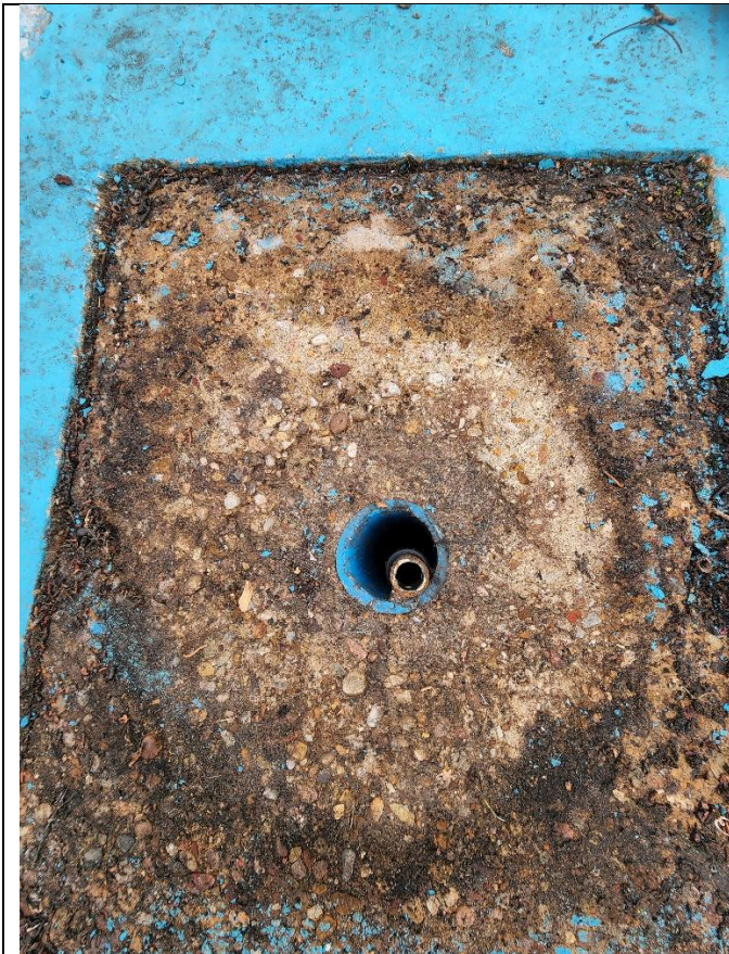
Photo 9: Central drain without cover over
