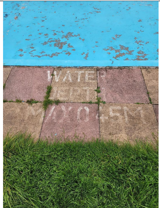
Photo 14: Painted markings to paving slabs - Faded
