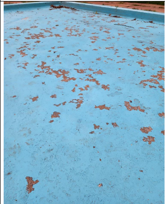
Photo 5: Delaminated paint throughout the pool tank
