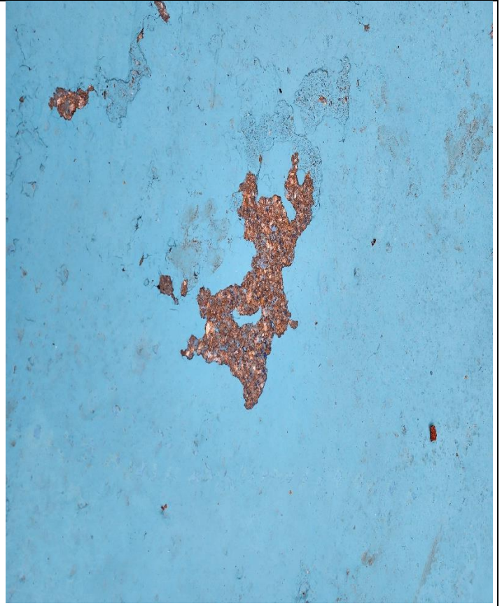
Photo 8: Example of paint delamination with screed below
