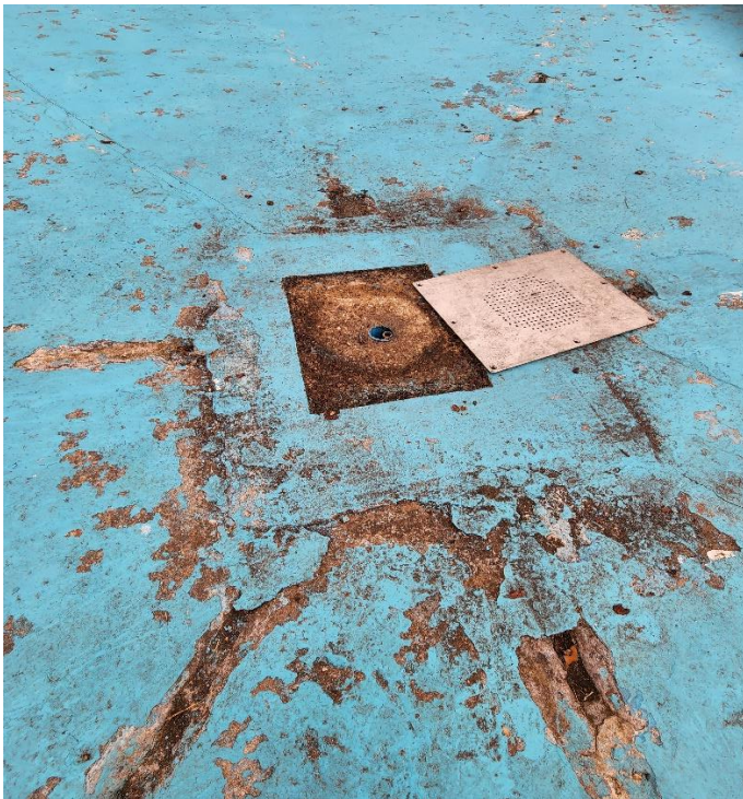
Photo 1 – Screed and Paint breakdown around drain
