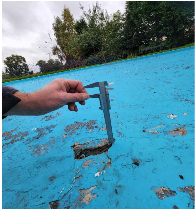
Photo 2 – Deepest Screed breakdown 20mm
