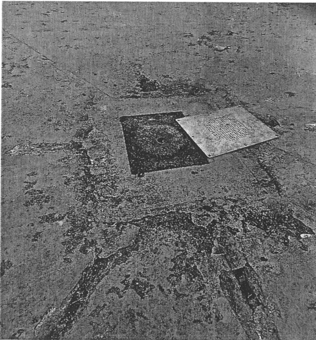
Photo 1 – Screed and Paint breakdown around drain
