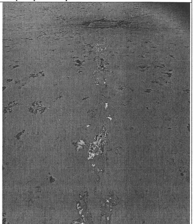
Photo 6: Pitting and delaminated paint example
