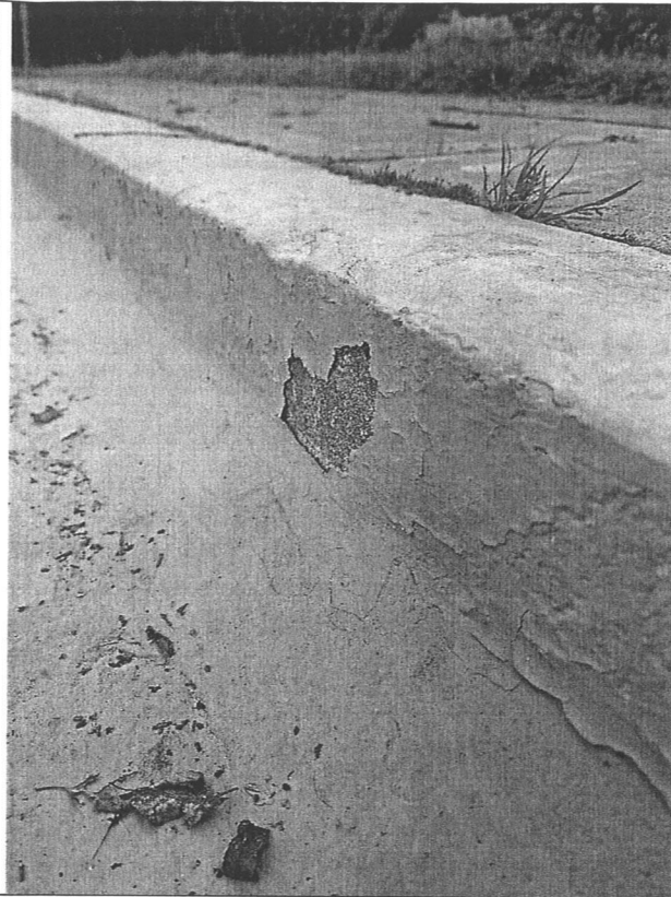
Photo 7: 1 isolated paint delamination to the upstand wall of the pool tank
