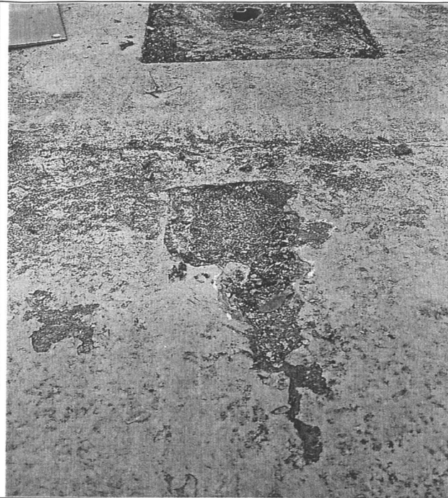
Photo 3: Further Screed breakdown
