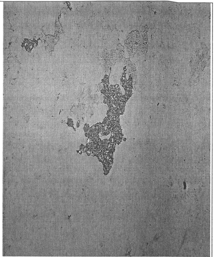
Photo 8: Example of paint delamination with screed below
