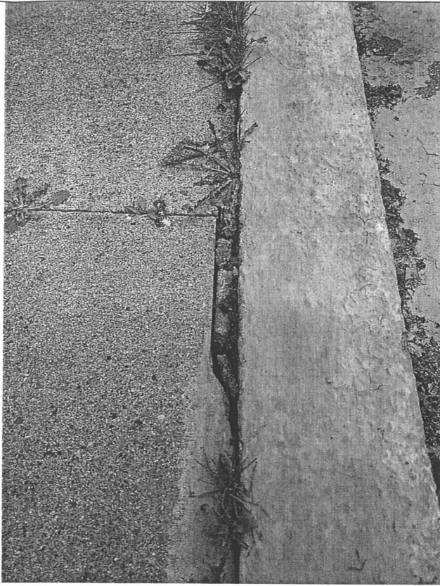
Photo 13: Missing pointing with vegetation growth
